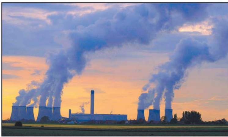
Dirty business... the UK's Drax Power Station which puts more CO 2 into the Earth's atmosphere than every car in England combined and burns 220 tonnes of coal every day. Picture: RICHARD CRAMPTON/REX FEATURES
