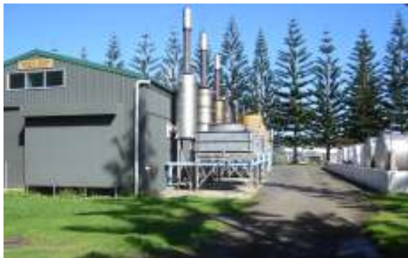
Fig. 10: Norfolk Island power house.
