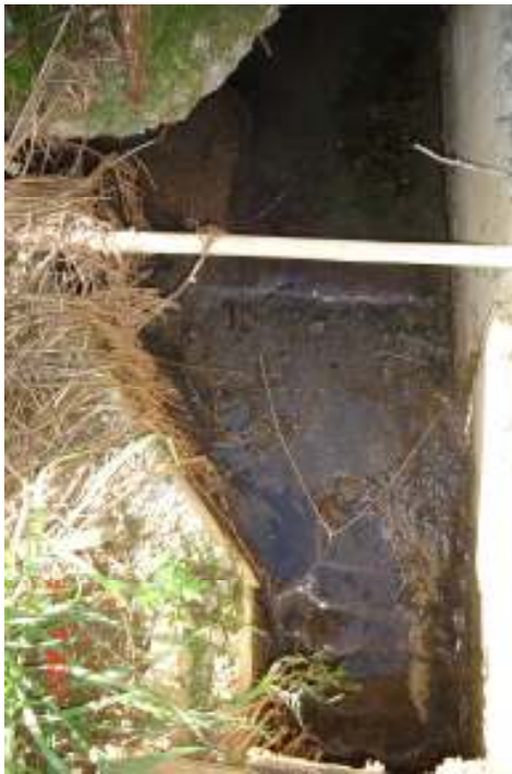
Fig. 7: One of many protrusions in channels connecting the pen pits with the digester.
